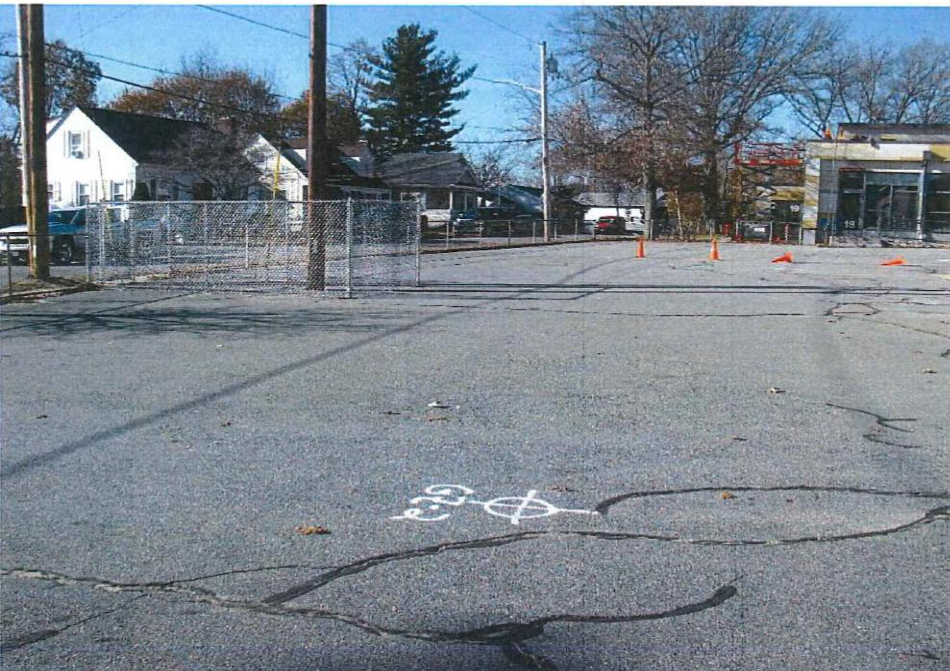
Photo 2 – View to west of existing paved play area (Gymnasium location)
