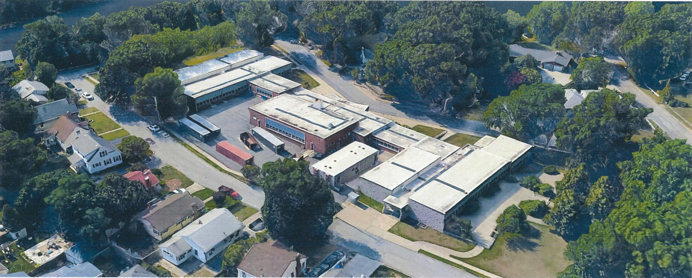
Aerial View – Chestnut Ave. Looking West
